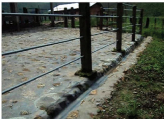
FIGURE 10.7: Stone Pavement Corral Floor at Munoh Farm
