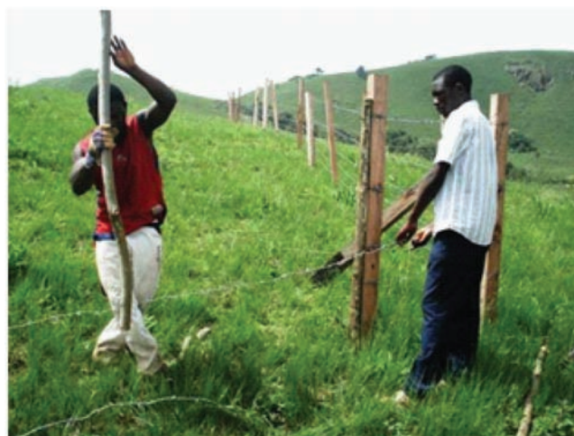
FIGURE 5.8: Constructing a Fence Gate
