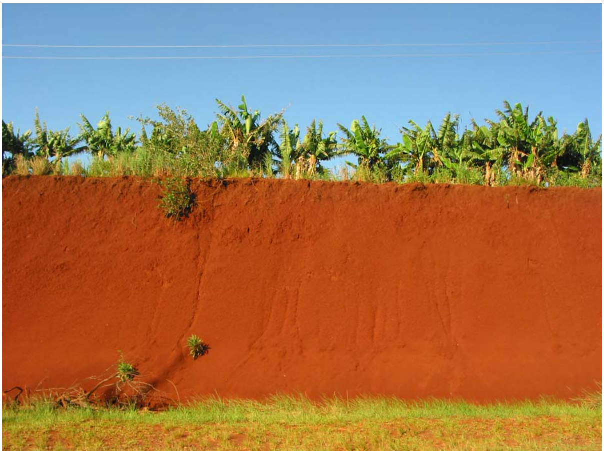
Figure 13. Lateral view in a rural dirt road in the Watershed of the Quiteria River, Itapua, Paraguay.
