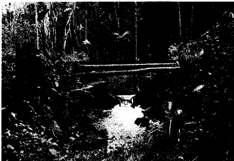
Fig. 3.3 Sharp-crested triangular weir for measurement of discharge; wet season
