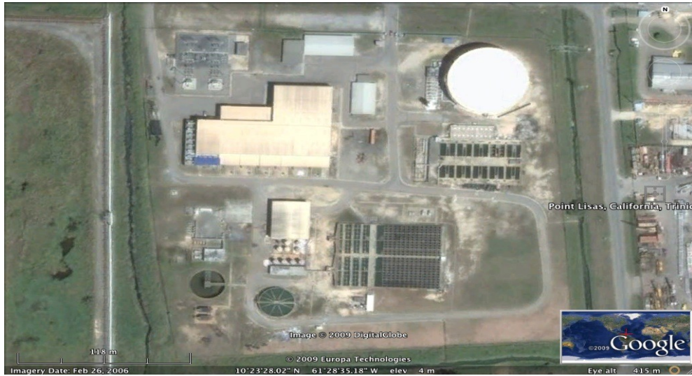
Figure 3.2 Point Lisas, Trinidad & Tobago SWRO Desalination plant (source: Google Earth February 26, 2006)
